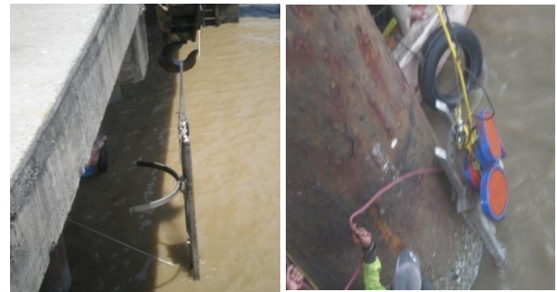
Fig. 6—Installation of Current Profiler
