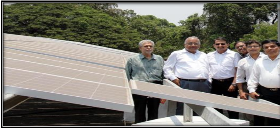
Fig 3.8 Solar Panel Installation
