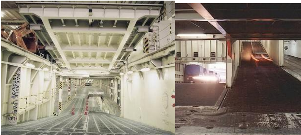
Fig15:Internal ramps usually which have 7° inclination.
