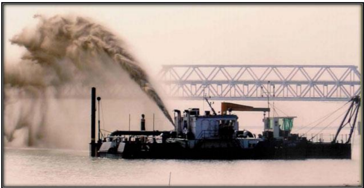
Fig 30: Dredging on National Waterway-1 is now underway.
