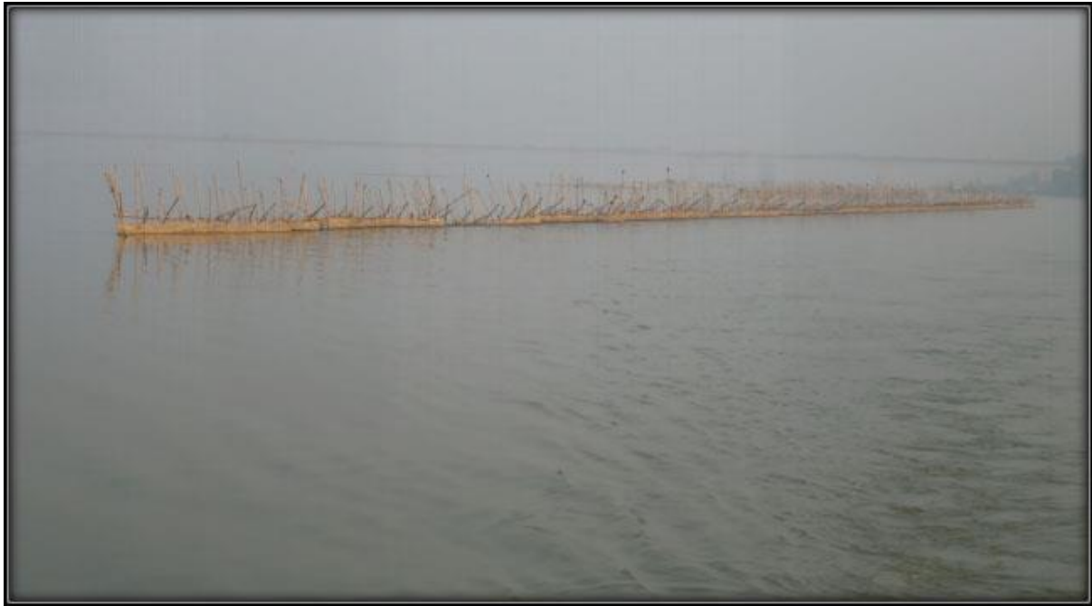
Fig 29: Along National Waterway-1, a bandal was erected.
