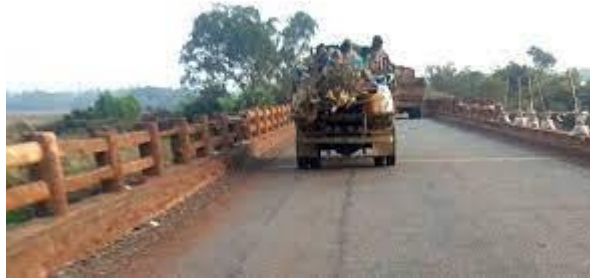
Survey Image of 6 Laning of NH-53
