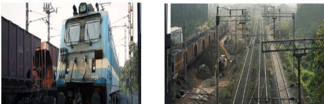
Railways Siding in Paradip Port
