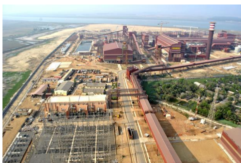
Conveyor System in Paradip Port
