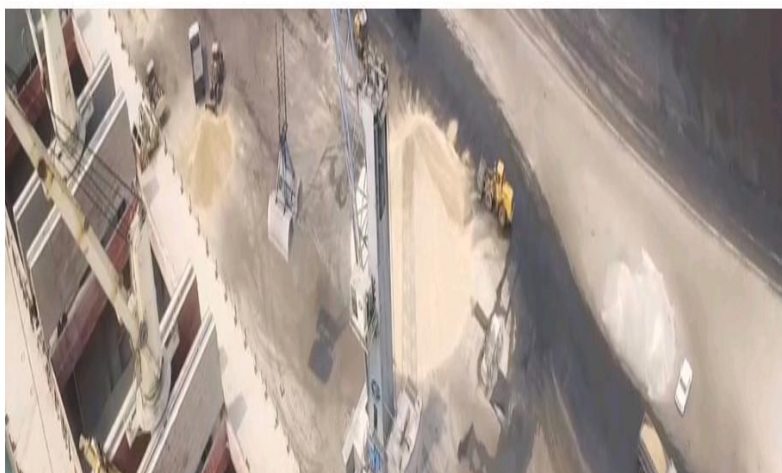
General Cargo Berth Paradip
