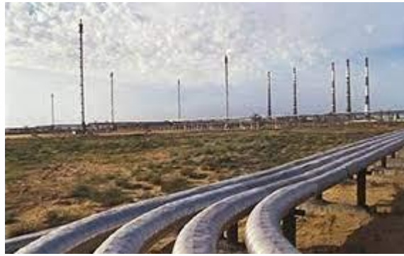
Paradip Hyderabad Pipeline Project
