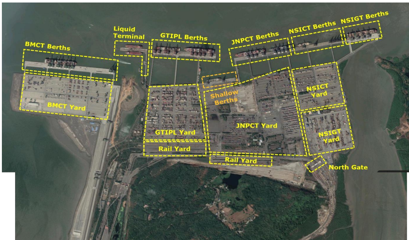
Figure : Existing Facilities at JNPT (retrieved from Google Maps)
