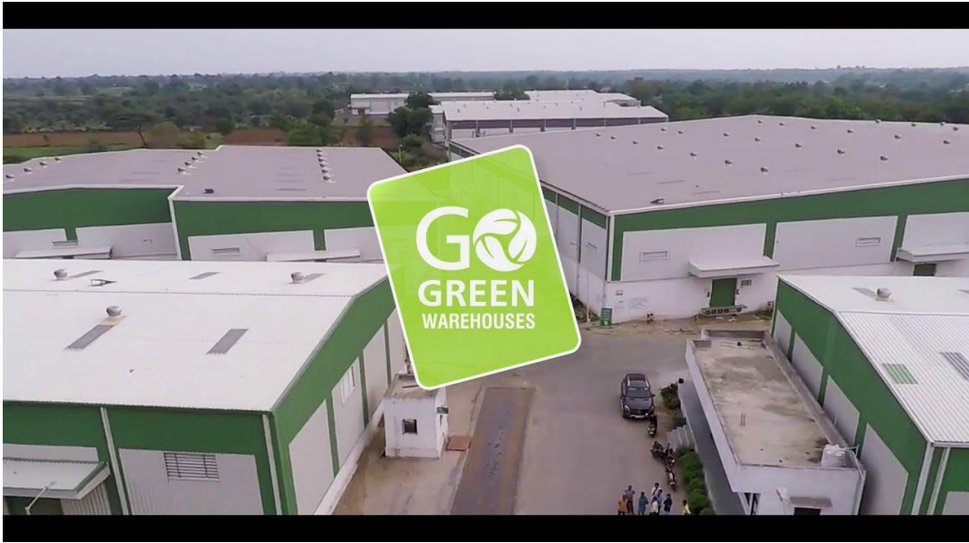
FIG 3.8 Go Green Warehouse
