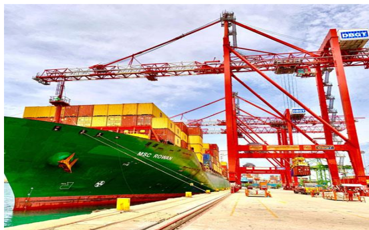
FIG 4.4 DAKSHIN BHARAT GATEWAY TERMINAL
