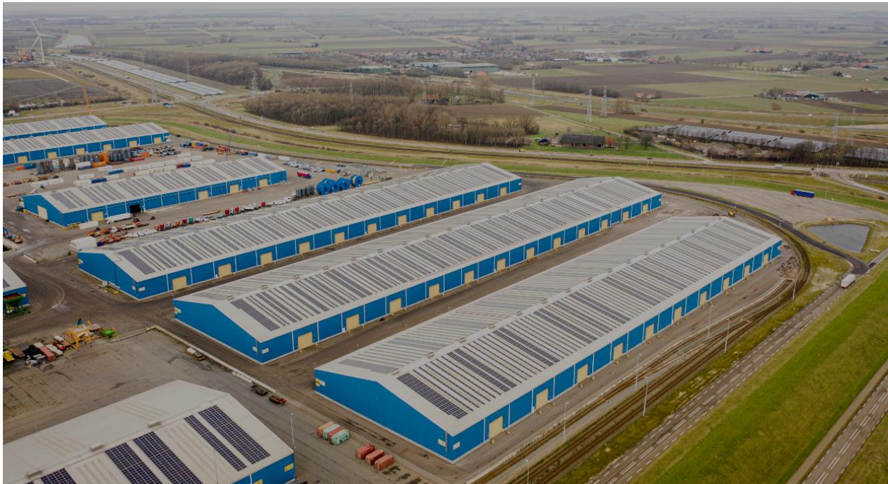
Fig 5.2 Solar Panel on Roof Top
