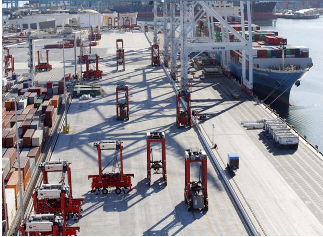
Fig 3.3 Automated Robot handling Container yard
