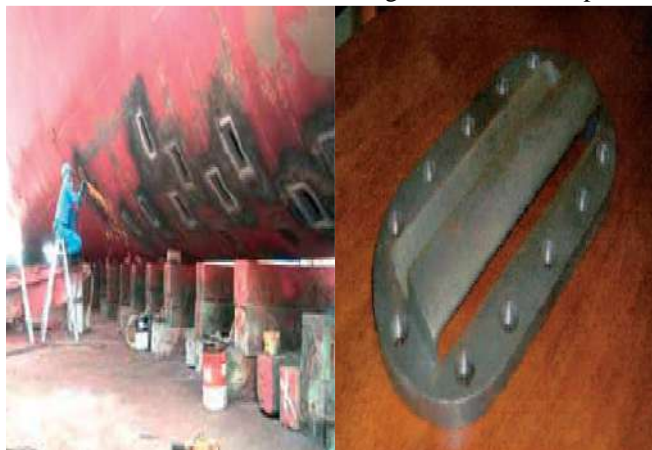
Fig. 2. WAIP installation process in dry dock and Cast iron WAIP fitting
