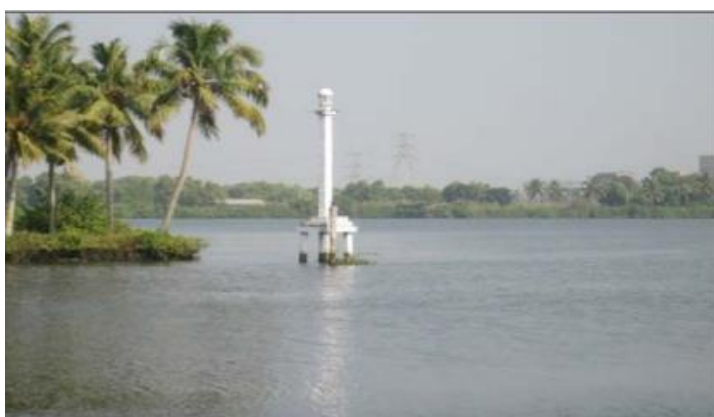
Fig 3.16 Beacon lamp in NW-3
