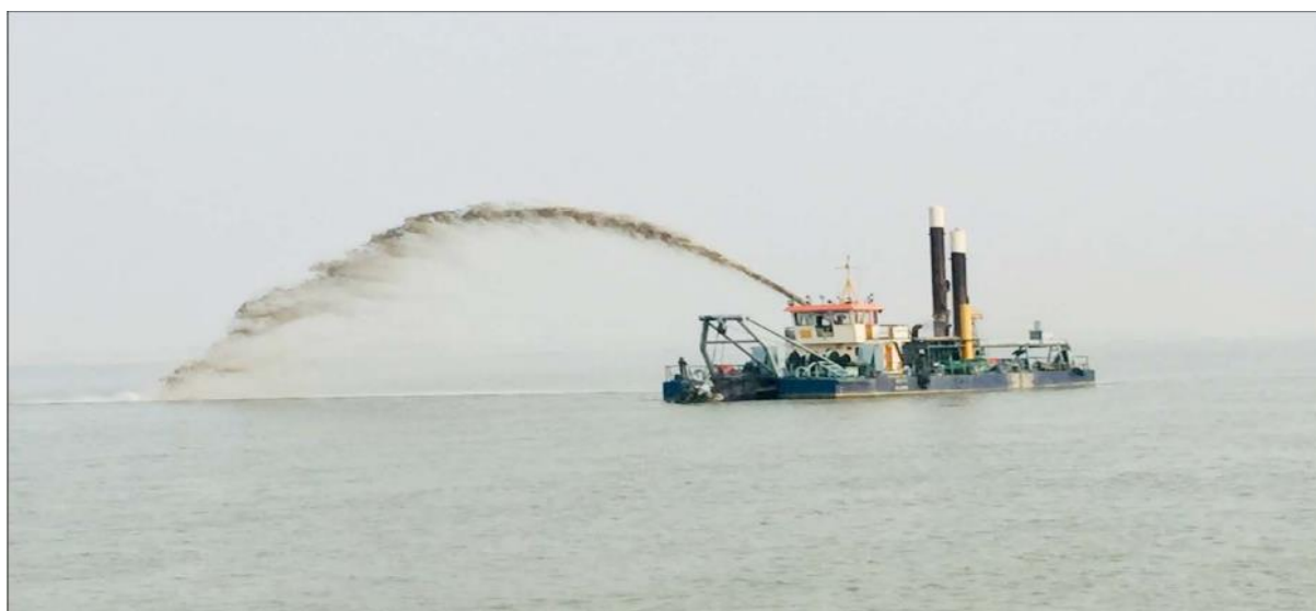
Fig 3.3 Dredging in progress on National Waterway-1
