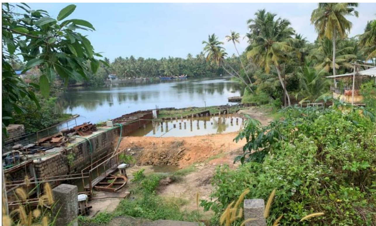
Fig 3.13 Piling work for Thrikkunnapuzha Lock construction is in progress
