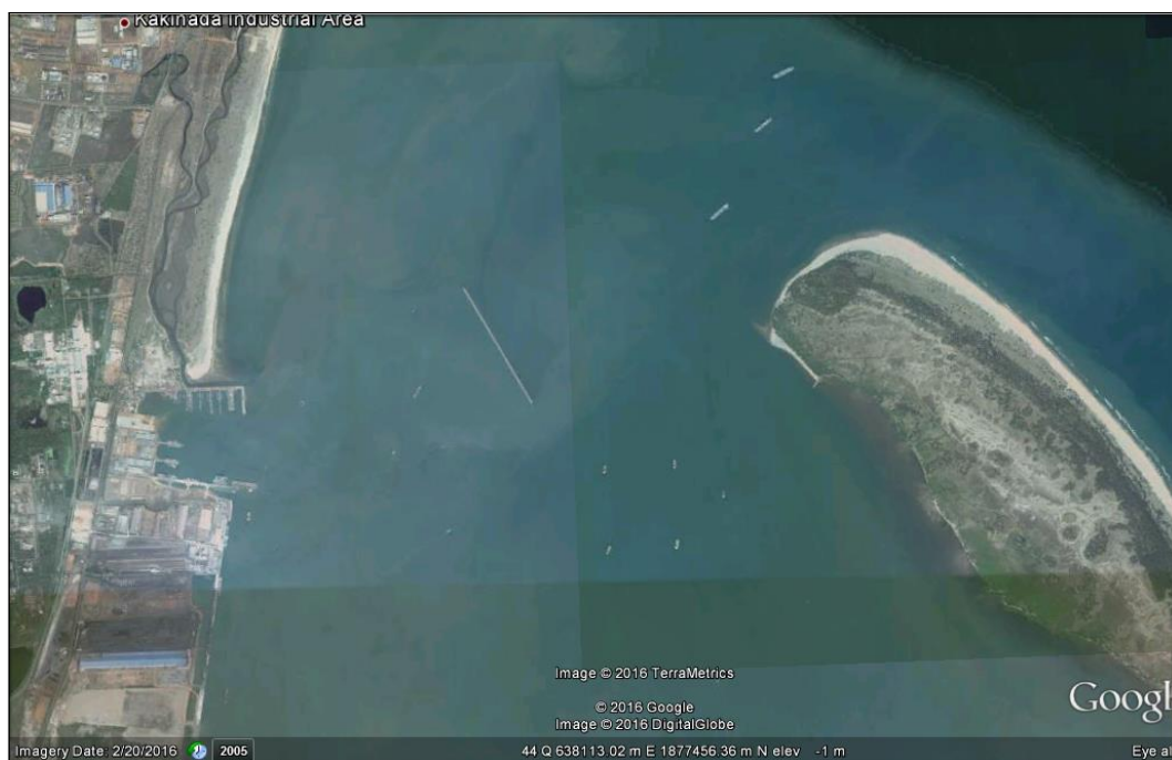
Fig. 3: Breakwater in Kakinada Bay (Source Google Earth).
