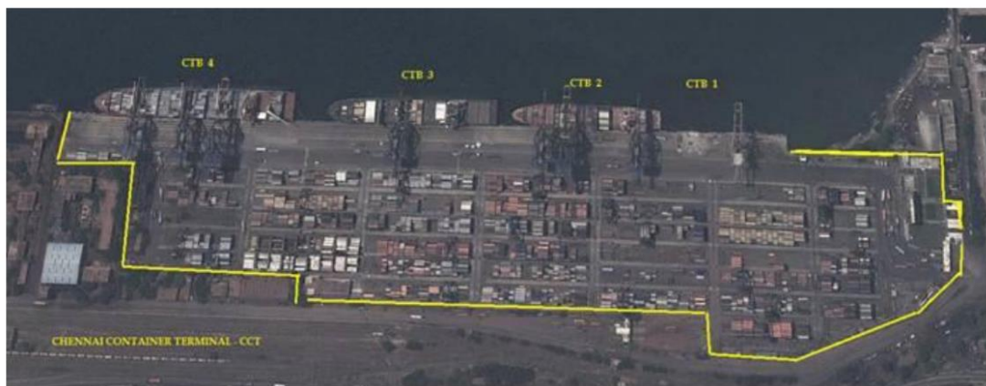
Figure 10: CCTL container terminal aerial view
