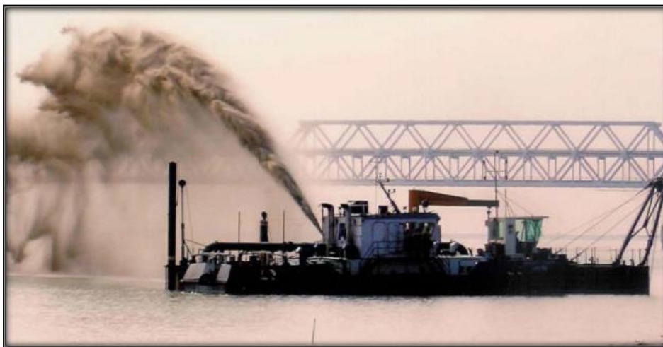
Fig. 2.2 Dredging in progress through the pipeline on National Waterway-1-
