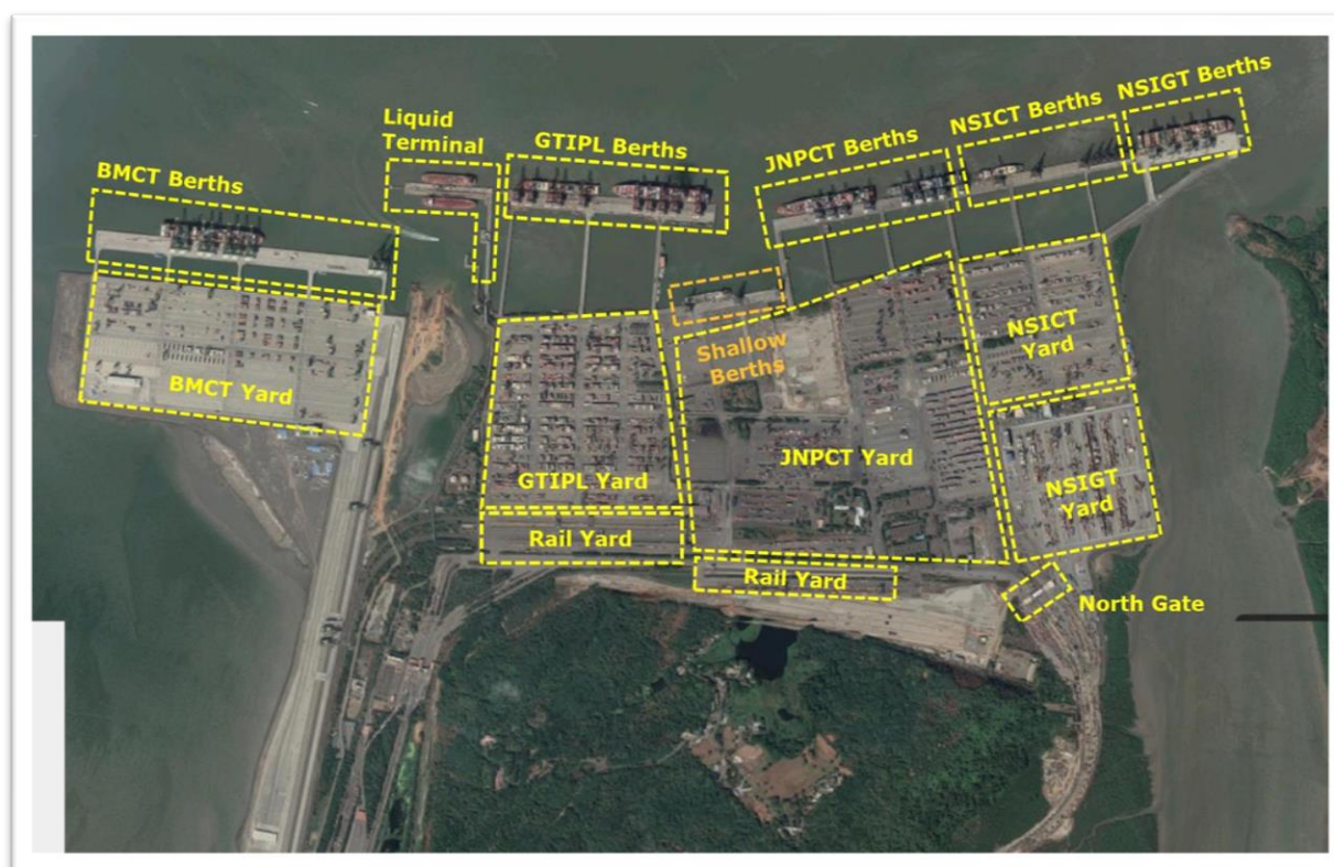
Figure 3.1: Existing Facilities at JNPT (retrieved from Google Maps)
