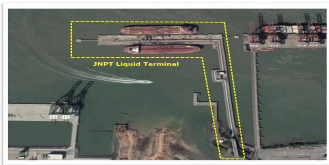
Figure 3.1.3: BPCL Liquid Terminal (retrieved from Google Maps)
