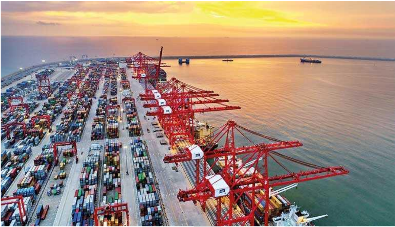
Colombo International Container Terminal
